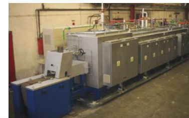
Powder metallurgy continuous sintering furnace
